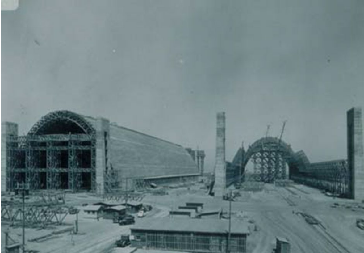
Photo 1: Hangars 2 and 3 Under Construction, 1943
